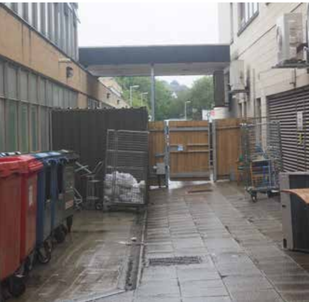
Figure 27 Light areas along back routes and alley ways from final exit doors. There is a break-glass exit release on the gate here
