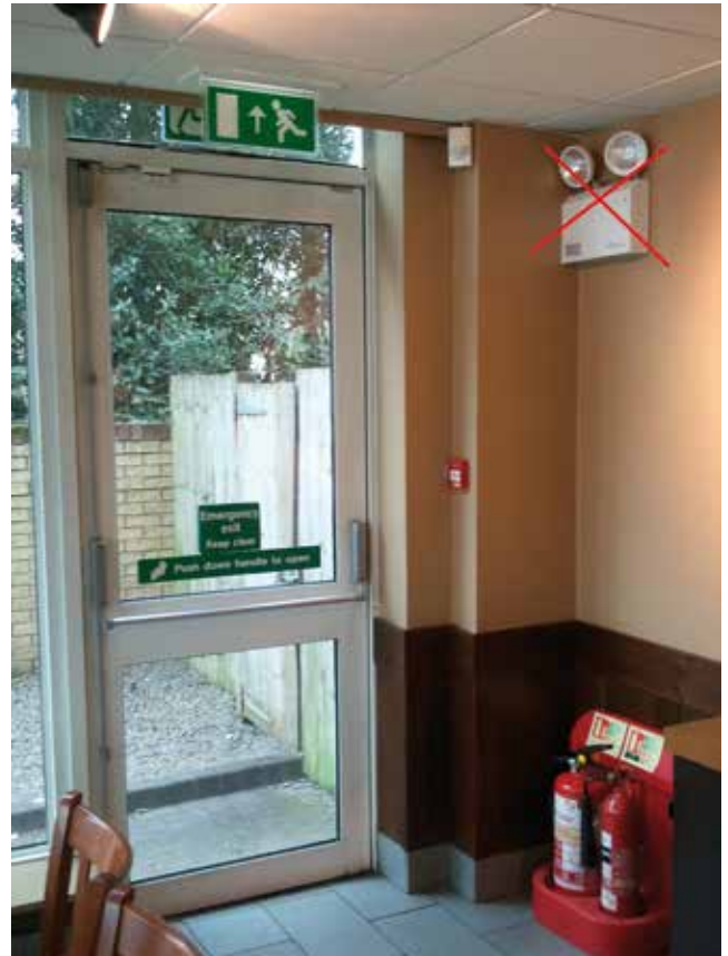
Figure 11 Do not place spot style lights at low-level or where they may dazzle escapees trying to find an exit
