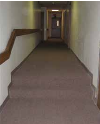
Figure 4 Ensure any junctions and isolated steps along escape routes are directly lit
