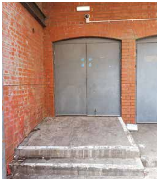
Figure 24 Exits with steps or slopes directly outside need to be well lit
