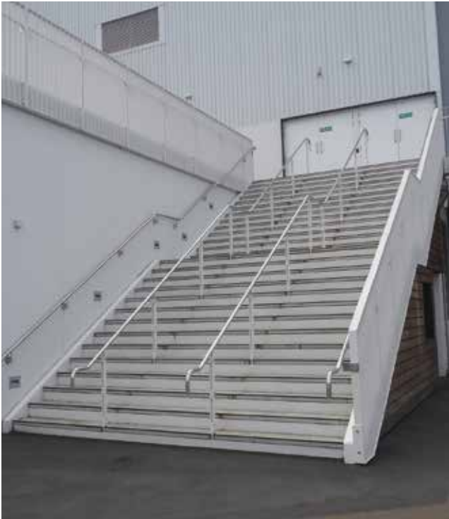
Figure 25 Continue emergency lighting and exit signage externally to a place of safety. All external stairways from exits need lighting
