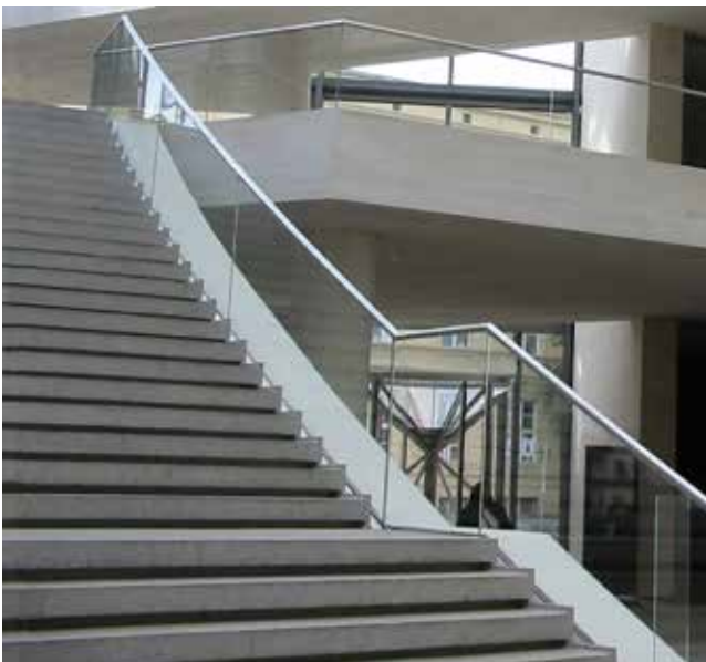
Figure 15 General access stairs should be covered even if they are not designated as escape stairs
