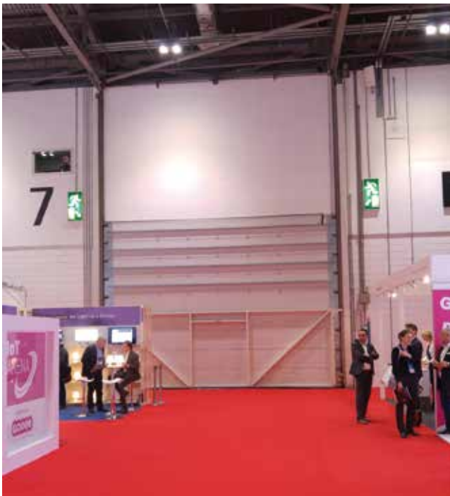
Figure 19 Check that exit signs are the correct size for their viewing distance. Large signs are available for big spaces
